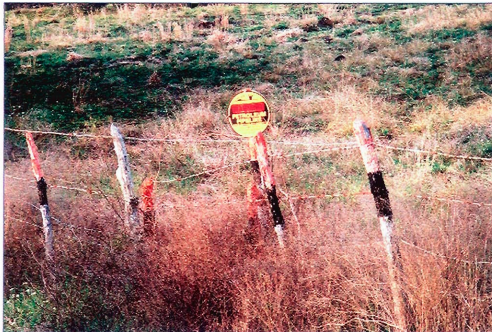
Figure 1: Poor markings and signage on out of use pipeline.
