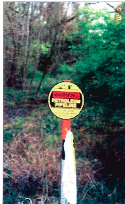
Figure 2: Right-of-way overgrowth, poor maintenance on 'idled' pipeline.
