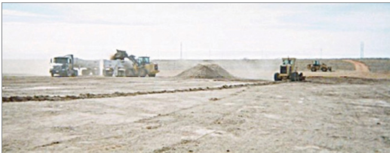
Grading location during final clearing.
