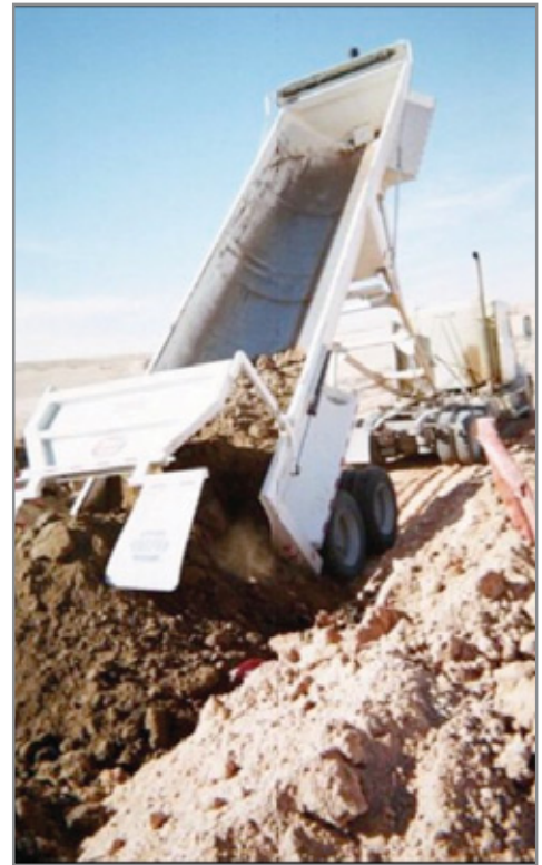
Surface soil right of way disposed of at landfill.
