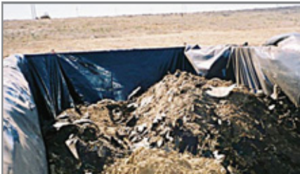
Coating and dirt loaded in lined container for landfill.
