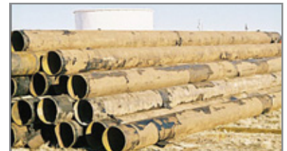
Coated pipes prior to cleaning.
